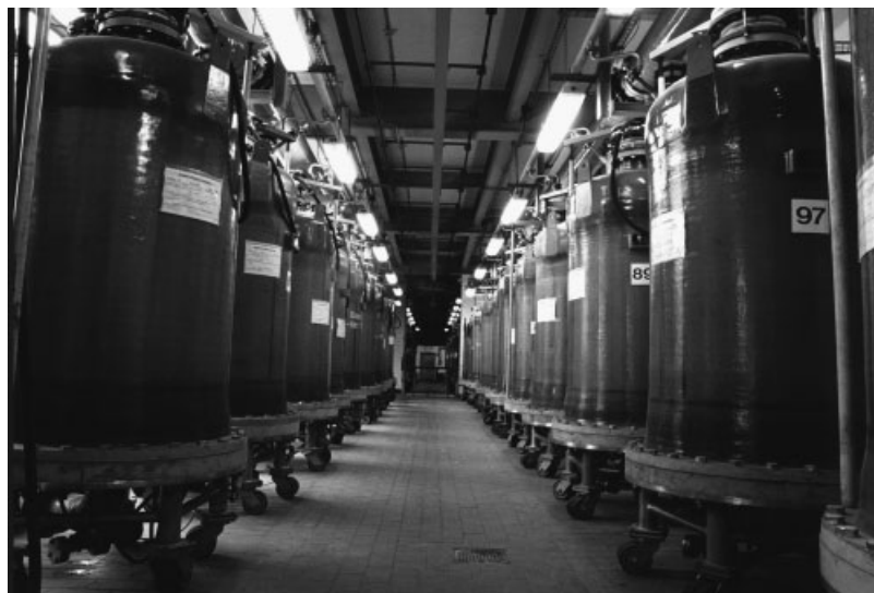
Fig. 7 Cell room with capillary gap electrolyzers [28] (photo: BASF AG).
